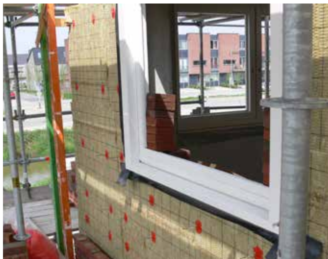
Prikspouwanker met UNI-CLIP
